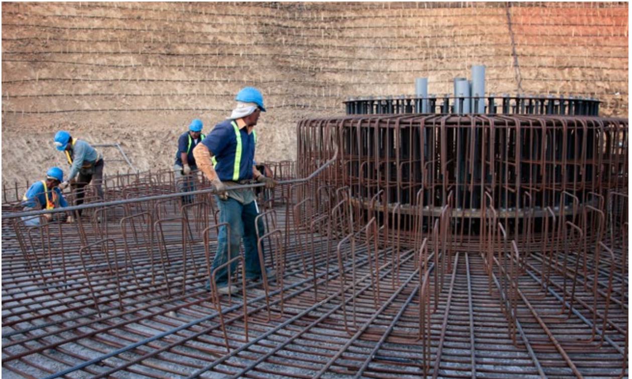
↑ Construction of a wind power generator (San Jose, Costa Rica)
