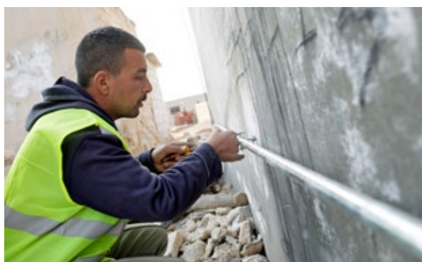
← Installation of drinking water pipes (Mafraq, Jordan)
